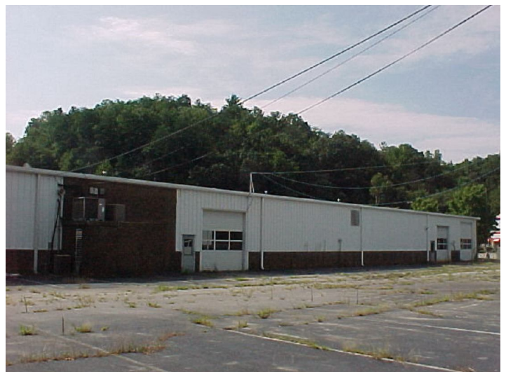
Rear of Building
